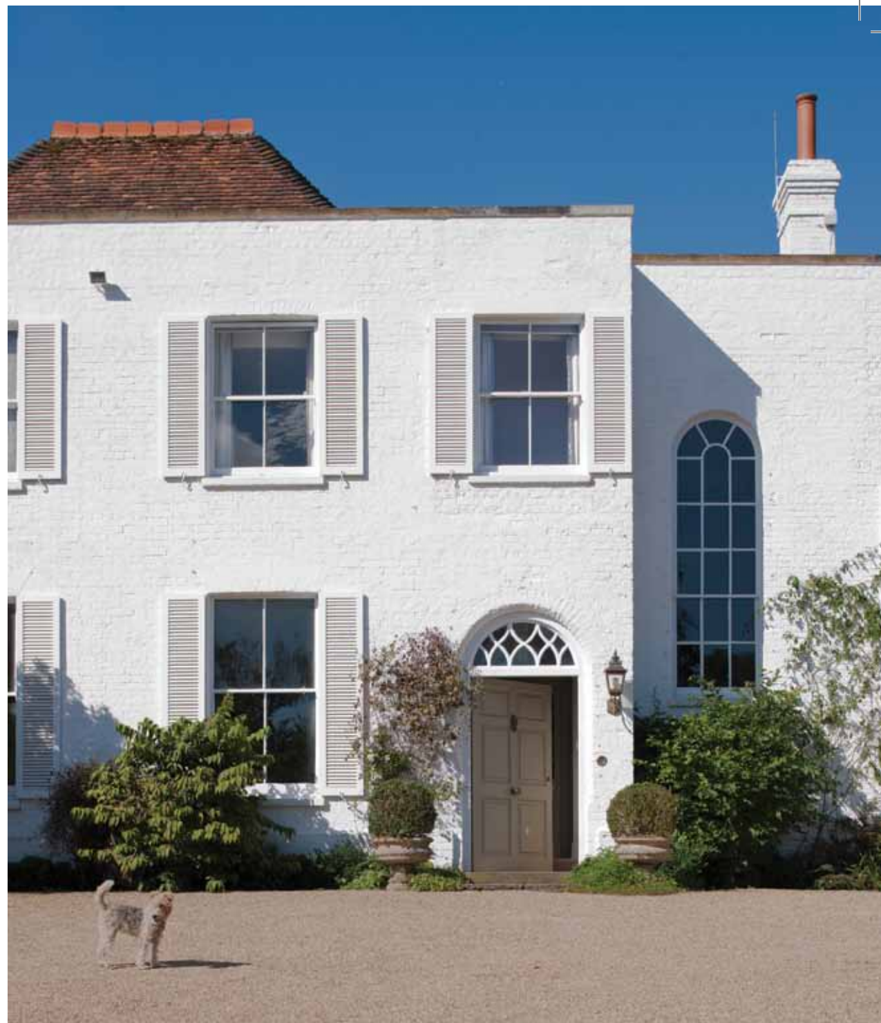
House: Wimborne White Exterior Masonry, Shutters: Wimborne White Exterior Eggshell, Door: Fawn Exterior Eggshell. 7
